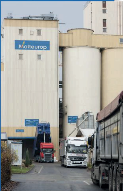
The European malt producer Malteurop uses Guntner air heater coils as well as thermowave plate heat exchangers in its refrigerating plant.
