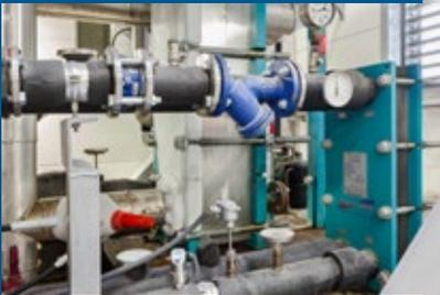
▲ A powerful thermowave NH<sub>3</sub> plate-type evaporator cools the glycol circuit for the supply of air coolers (back) and another thermowave plate heat exchanger (front) supplies the centralised ventilation system for the offices.
