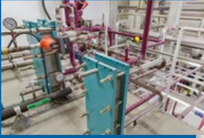
▲ The waste heat from the NH<sub>3</sub> evaporator is transferred via thermowave plate heat exchangers to glycol circuits. The waste heat is used to heat the offices and the foundations in order to ensure that the ground underneath the storage room always remains frost-free, hence preventing the floor slab from suffering any structural damage.
