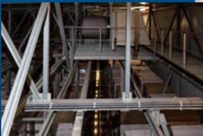
▲ The nine Güntner HIGHSTORE Application air coolers in the deep-freeze storage room sit 36 m/118 ft high, above the top edges of the racks, on a stage.
