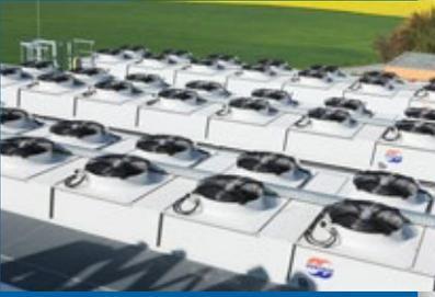
▲ AGVH-type Güntner FLAT Vario condensers each with 595 kW/2,030 MBTU/h have been designed as special units due to building regulation noise specifications of 50 dB(A)/10 m (33 ft) in order to achieve the specified operating parameters.
